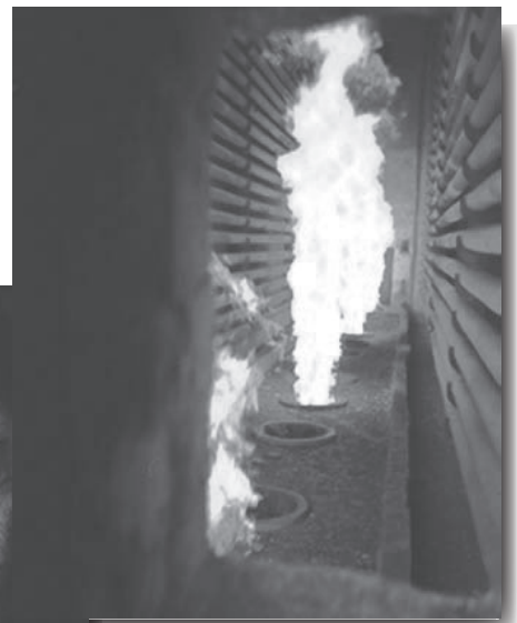
Gas Burner in Fire Box
